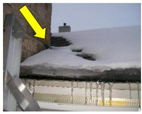
When the roof shingles were installed the were not hung over to allow the rain water to drip into the guer. This can cause water to get behind the shingles. This should be sealed and maintained.
