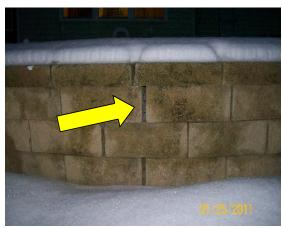
The Blocks appear not to have been secured. I also did not see a drain that would minimize water damage.
