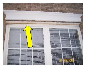
Here is another ice dam. There is also evidence of home owner repair. The use of roofing tar against the home where the shingles meet and around the corner are evidence of water intrusion.
