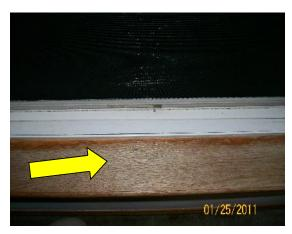
There is apparent water damage on the some of the second story window sills.
