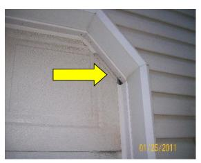
There are missing vents that cover the dryer exhaust. There is not a dryer attached hence the rag to stop the air flow.
