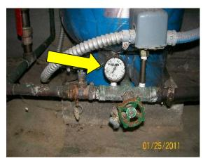
The incoming water line and electrical line to the water pump were cemented in to the wall.
