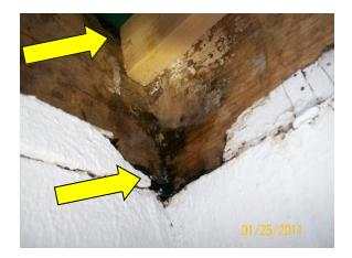
This is a second picture showing that the header is actually missing.
