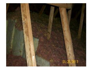
As I moved some of the insulation from the vertical exterior wall there is apparent mold growth. This should be tested and an mold inspection ordered.
