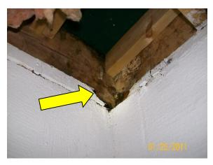
Here is some additional water damage on the header.
