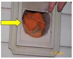
This is an unusual exhaust vent for the furnace. It causes excess water on the window above.
