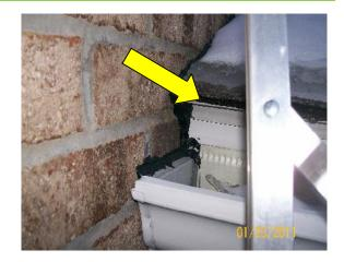
This is a big problem that needs to be repaired. The water form another secon of the roof is dump ing on the a lower roof. Shingles were not designed to stop this much water. If this is not leaking now it will.
