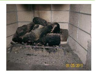
On Gas fire place has a lot of black ash or soot that I would not expect. This appears to say the gas logs are not burning correct. This should be checked replaced.
