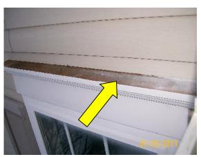
The white ash like substance is where the paint used is washing o and on to the window.
